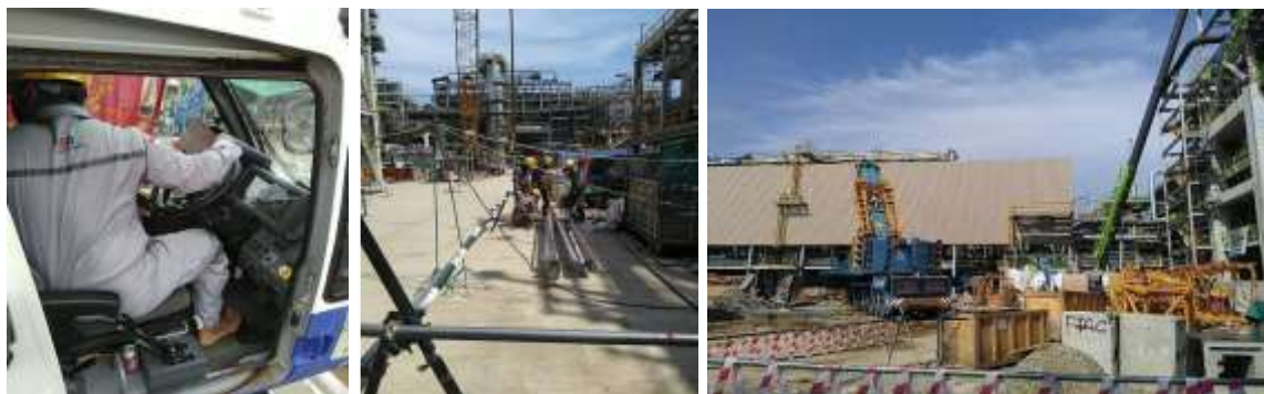
c) Lifting Activities by Crane Operator
