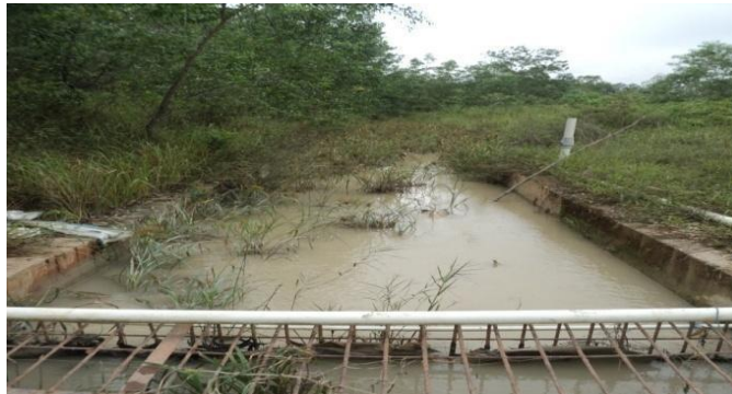
Gambar 8. Treatmend Pond Sumber: PT Adaro Indonesia, 2022
